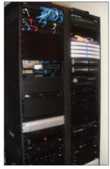
The Smart-e SNX-8x8+ was chosen for the project. Located in the hub of the house, the SNX-8x8+ delivers High Definition (HD) video to eight display screens around the property. All the sources are routed into the Smart-e SNX-8x8+ which are then scaled up to 1080p before they are switched through to the various rooms -
