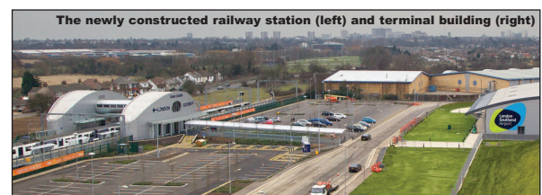
The newly constructed railway station (left) and terminal building (right)
