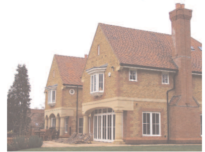
2 newly constructed multi-million pound properties nestled in the English countryside feature Smart-e equipment
